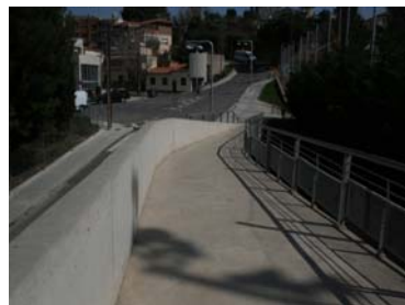
Rampa 2. Tram superior
